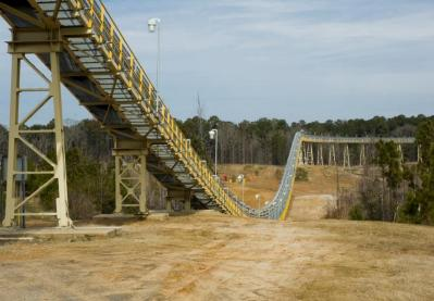
1.5 mile conveyor1.5M tons of pet coke by barge
