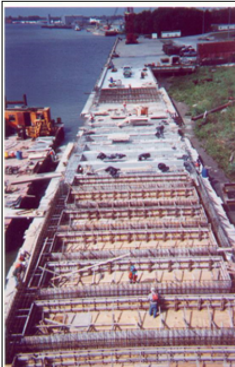
Figure 3 Workers building the East Dock Extension in 2000. Notice that it does not extend to the levee like the original wharf in the background. Photo courtesy of GSE and Associates, Inc.
