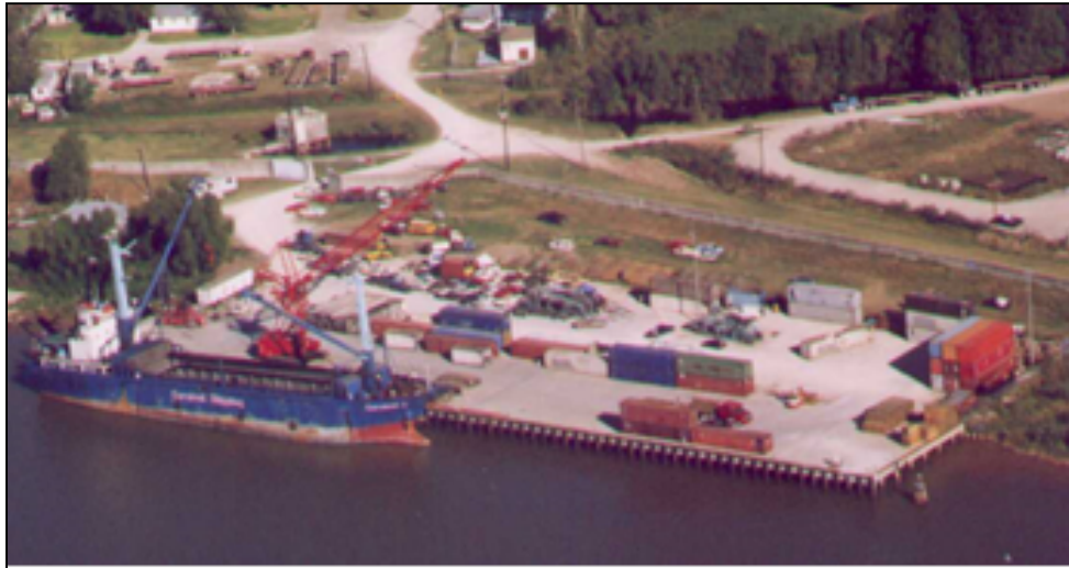
Figure 2 Original wharf in use following its completion in 1995. Photo courtesy of GSE Associates, Inc.
