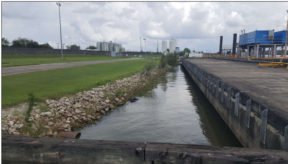
Figure 15 Photo of area of Eastern Enhancement project site where current dock (on right) will expand to the left onto the land and build a concrete cargo-handling area.
