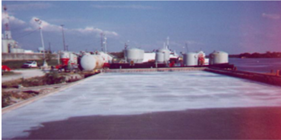
Figure 5 The East Wharf Extension completed in 2000. Photo courtesy of GSE and Associates, Inc.
