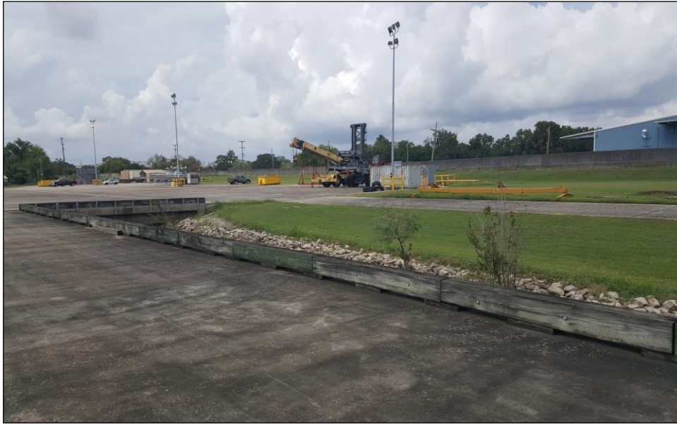
Figure 6 The FY 2017 TIGER Grant will fund a replication of the current dock and concrete apron (background) on the Eastern (foreground) and Western (not shown) sections of the port's dock.
