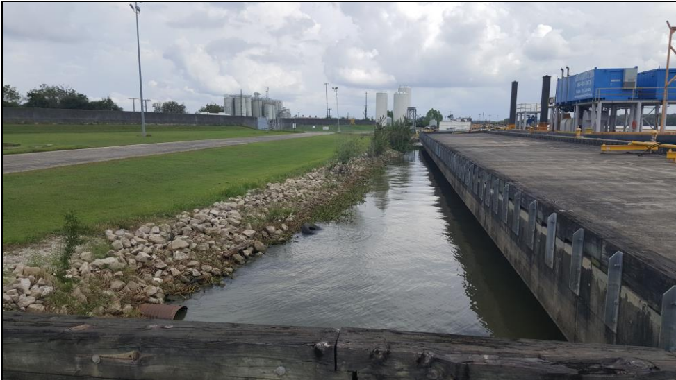
Figure 3 Photo of area of Eastern Enhancement project site where current dock (on right) will expand to the left onto the land and build a concrete cargo-handling area.
